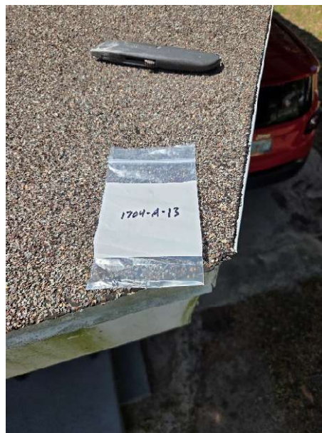
Sample 1704-13 Typical Rolled Asphalt Roofing Sample
